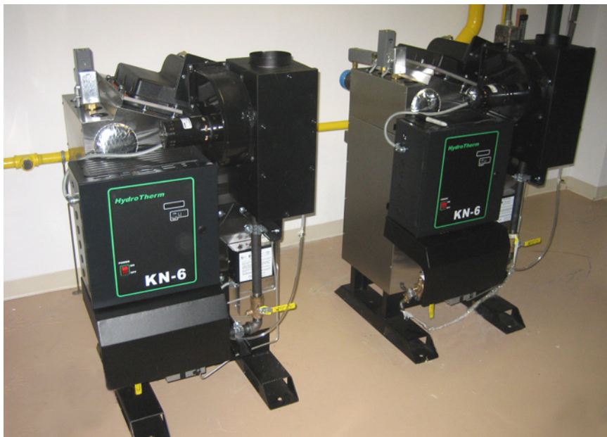
KN-6 boiler installation at One Corporate Place, Danvers, Massachusetts
