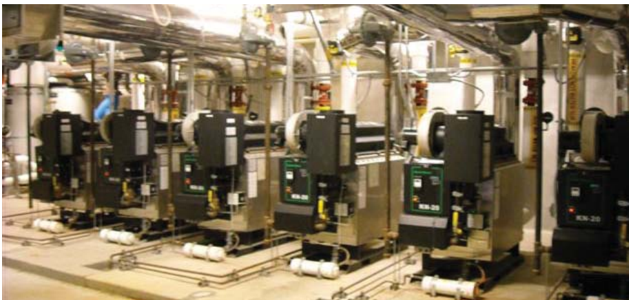
Newly installed, this system of six interconnected, fully condensing KN-20 boilers is ready to go into operation.
